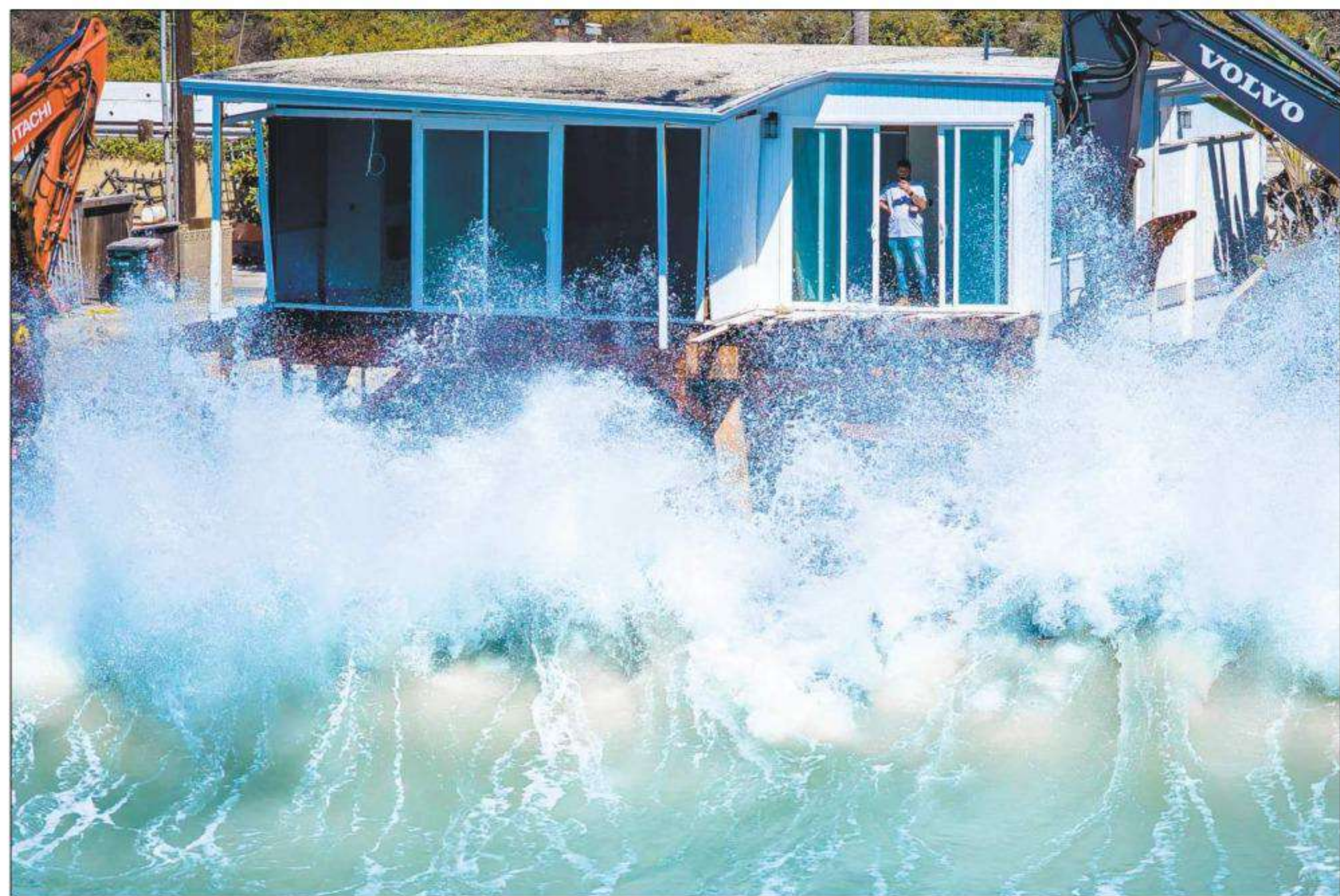
HEAVY machinery moves boulders into position to reinforce a seawall in Capistrano Beach on Tuesday.
